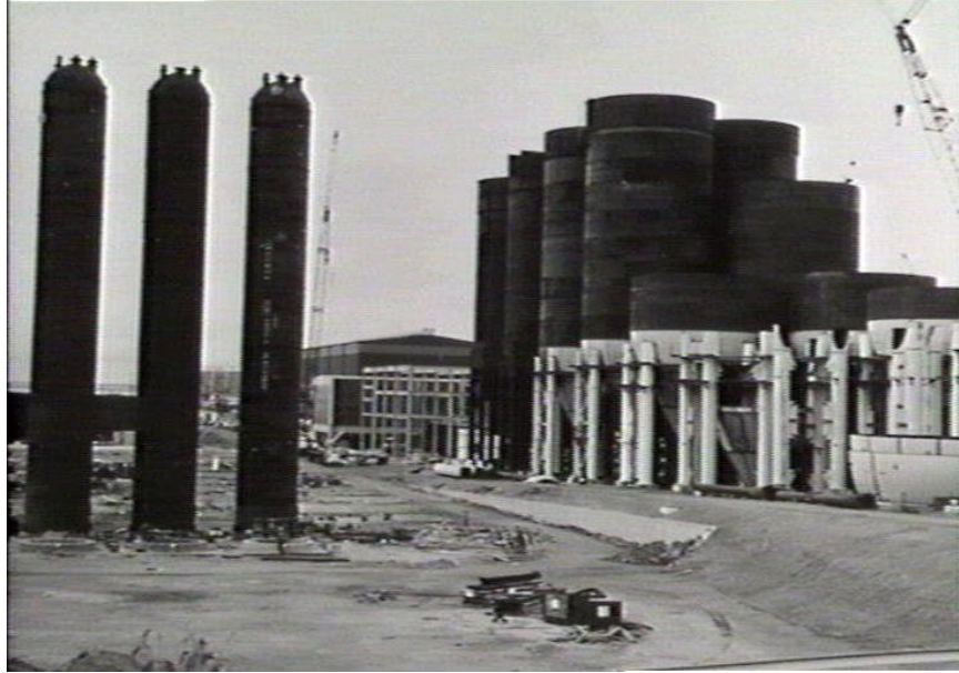
Figure 9. The Gove alumina refinery under construction, 29 January 1971. Photograph: M. Willmott. Northern Territory Government Photographer Collection, Library & Archives NT, PictureNT PH0095/0046, https://hdl.handle.net/10070/721531 . Licensed CC BY 4.0.
