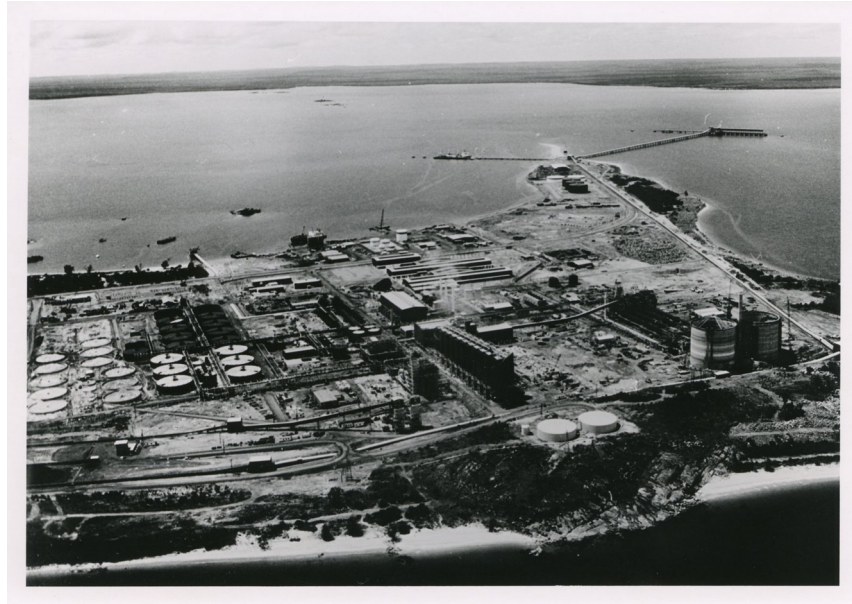
Figure 5. Aerial view of the Nabalco plant site, Gove, 26 February 1970. Photographer not recorded. T. N. Renton Collection, Library & Archives NT, PictureNT PH0142/0020, https://hdl.handle.net/10070/750758 . Licensed CC BY 4.0.
