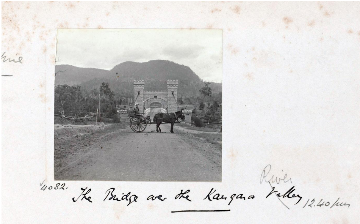
Image 3 One of the earliest photos of Hampden Bridge circa 1899/1900 Album 24: Photographs of the Allen family, 14 November 1899 - 4 November 1900, PX*D 569, 26l4xBq4GPr23
