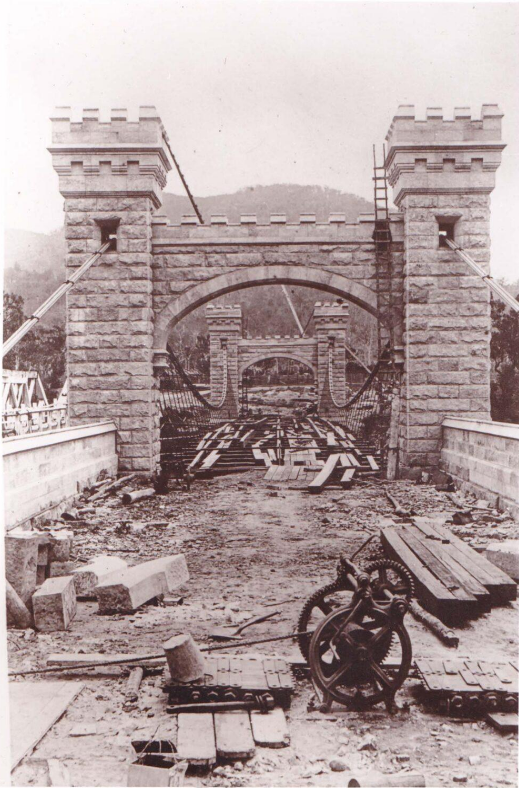
Image 10 Hampden Bridge Construction 1897/8
