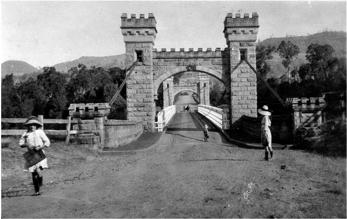
Image 5 Hampden Bridge, Suspension bridge - Kangaroo Valley, NSW, c 1910, SLNSW nQRBvNA1
